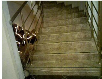
Figure 8. Spiral staircase (colour image)
